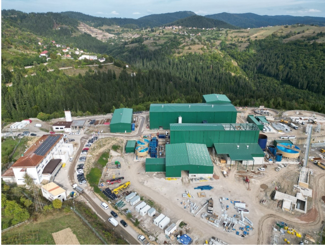
Figure 7: Aerial view of the Vares Processing Plant, September 2023
