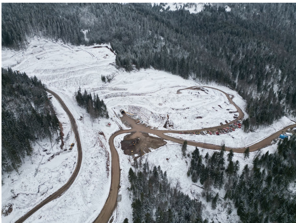
Figure 3: Upper Decline Portal
