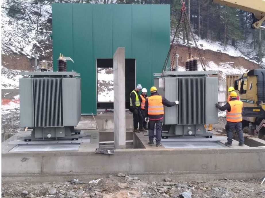
Figure 1: Rupice Transformer installation
