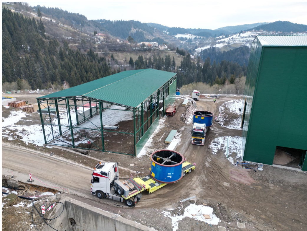
Figure 7: Oversized delivery of mill at VPP
