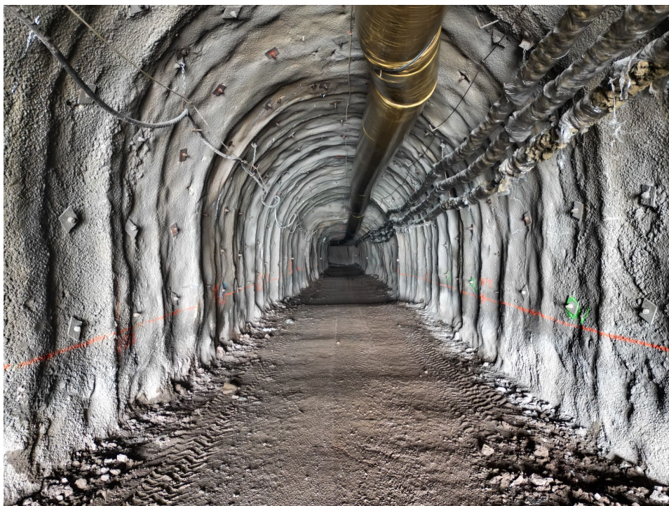
Figure 2: Underground at the Upper Portal
