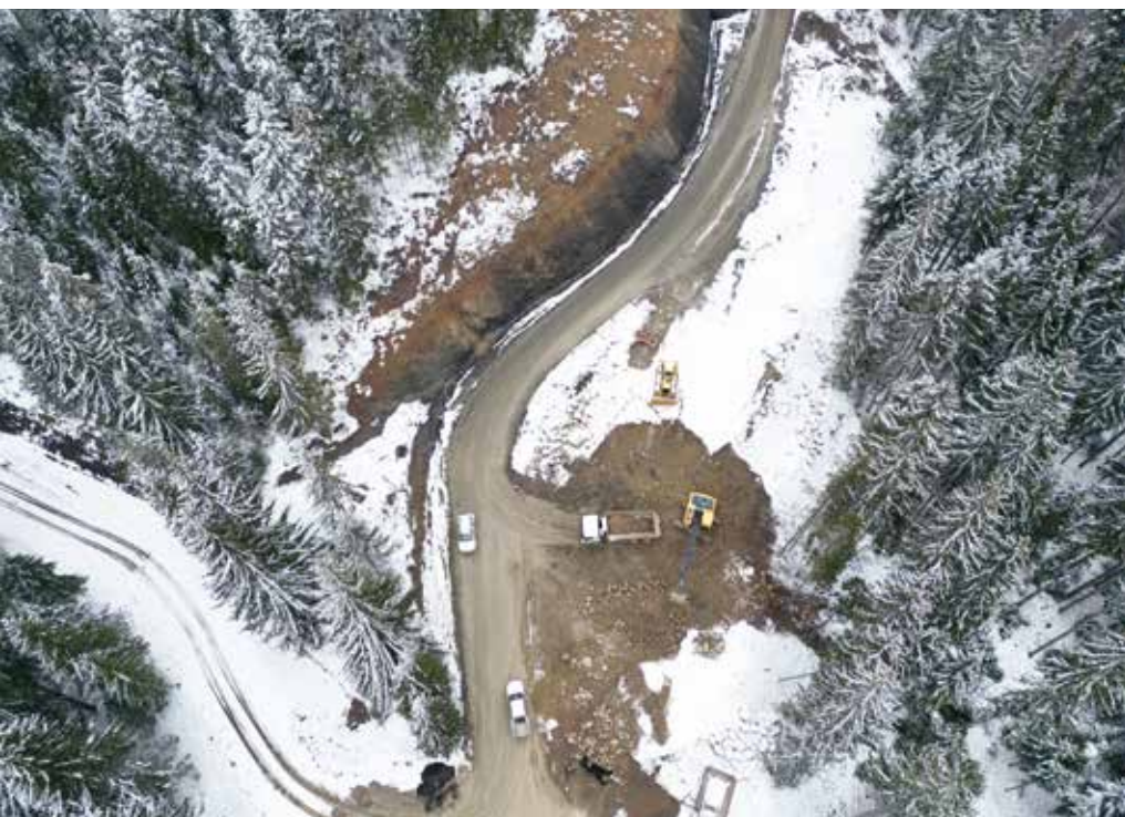
The 24.5km haul road remains on schedule for completion next quarter
