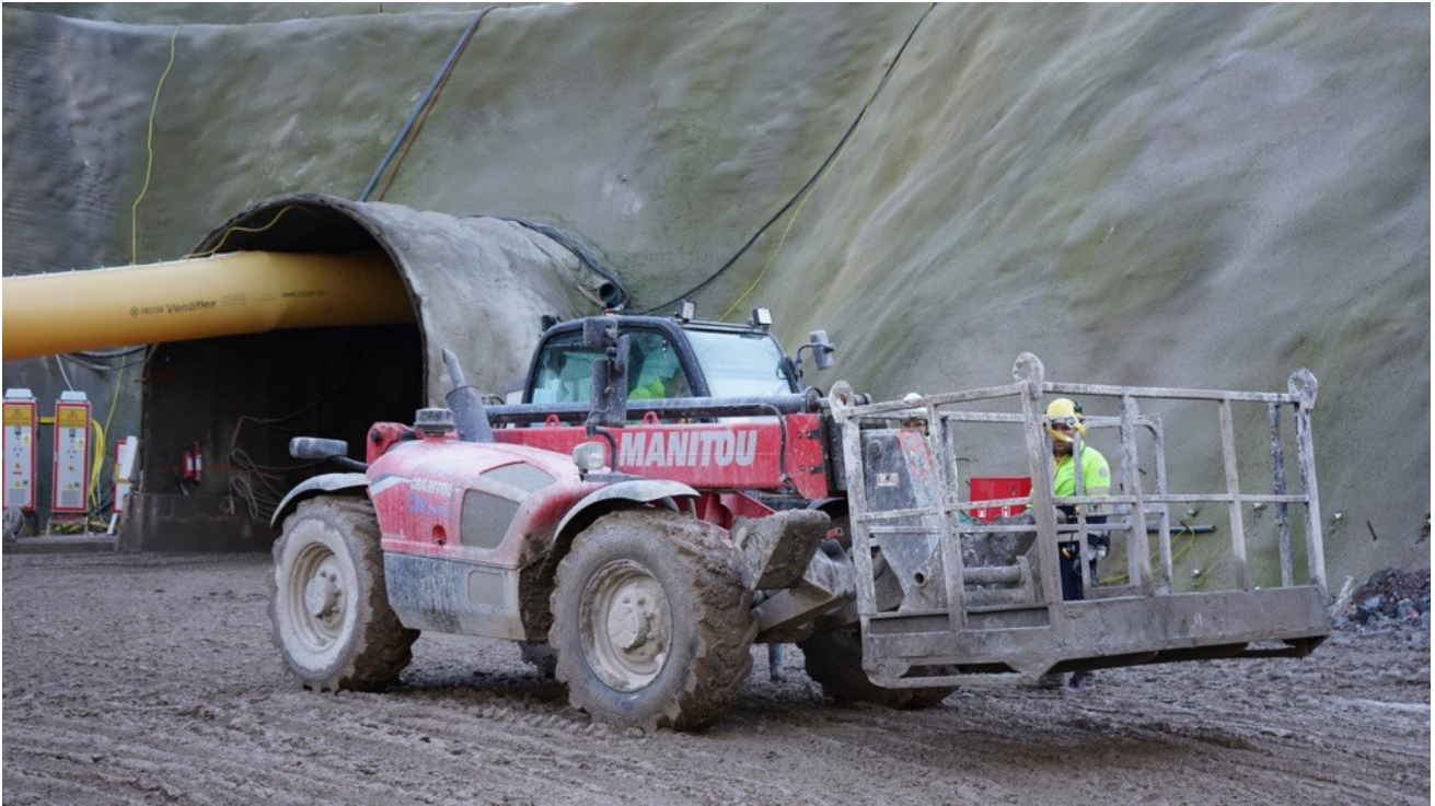
Figure 3: Lower Decline Portal
