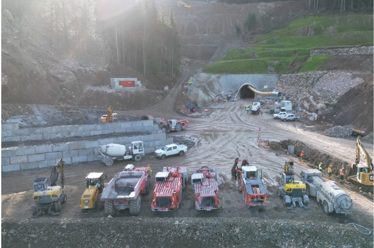
Figure 1: Lower Decline Portal
