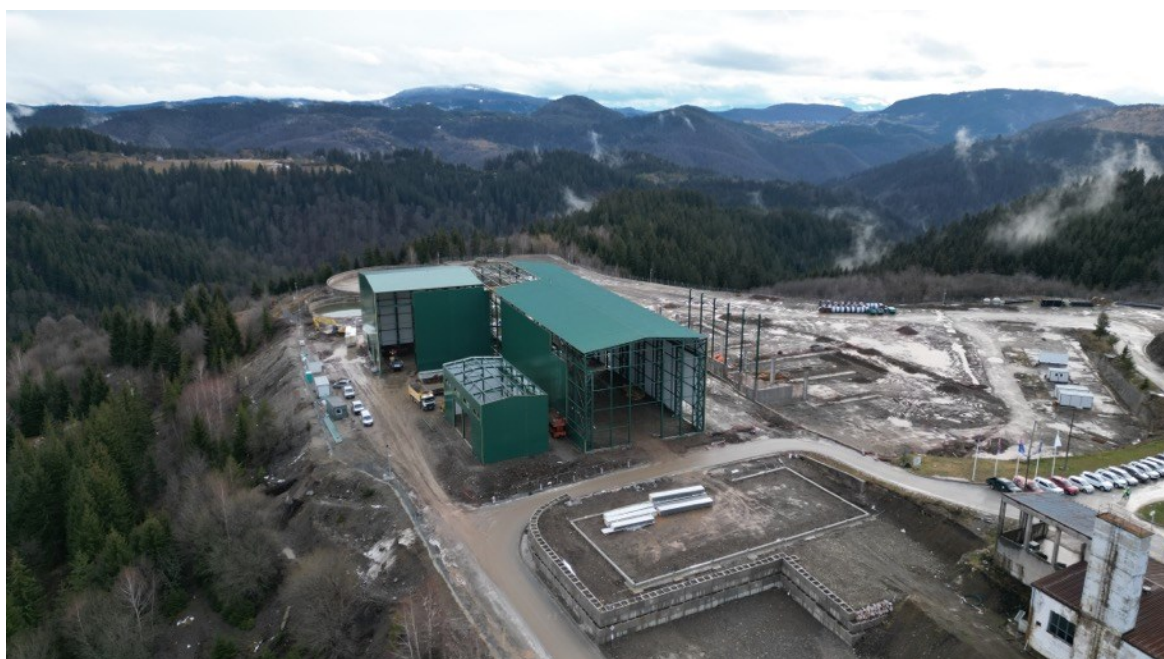
Figure 5: Vares Processing Plant
