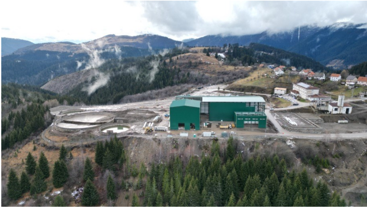
Figure 6: Vares Processing Plant
