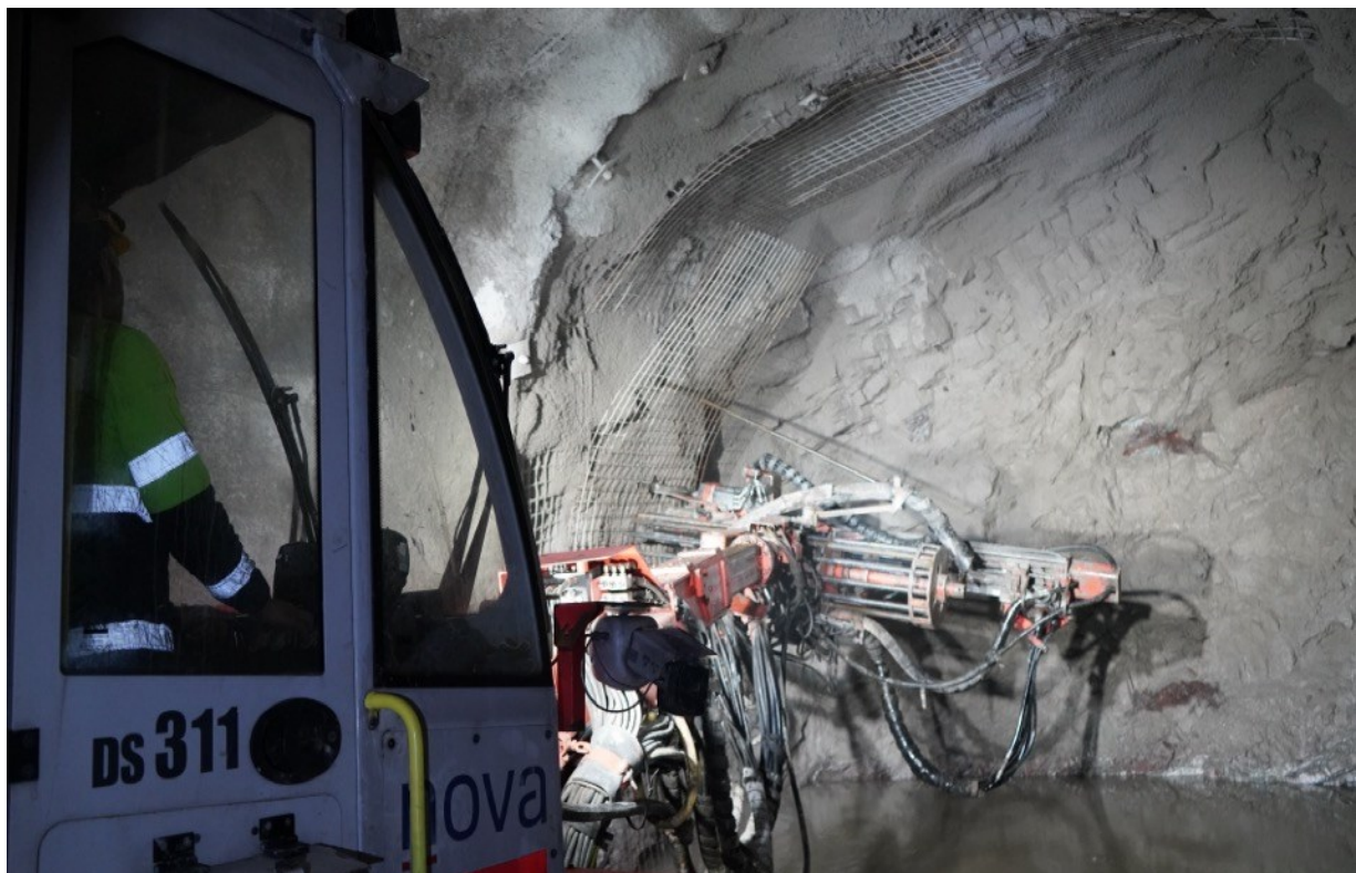
Figure 2: Underground at the Upper Portal
