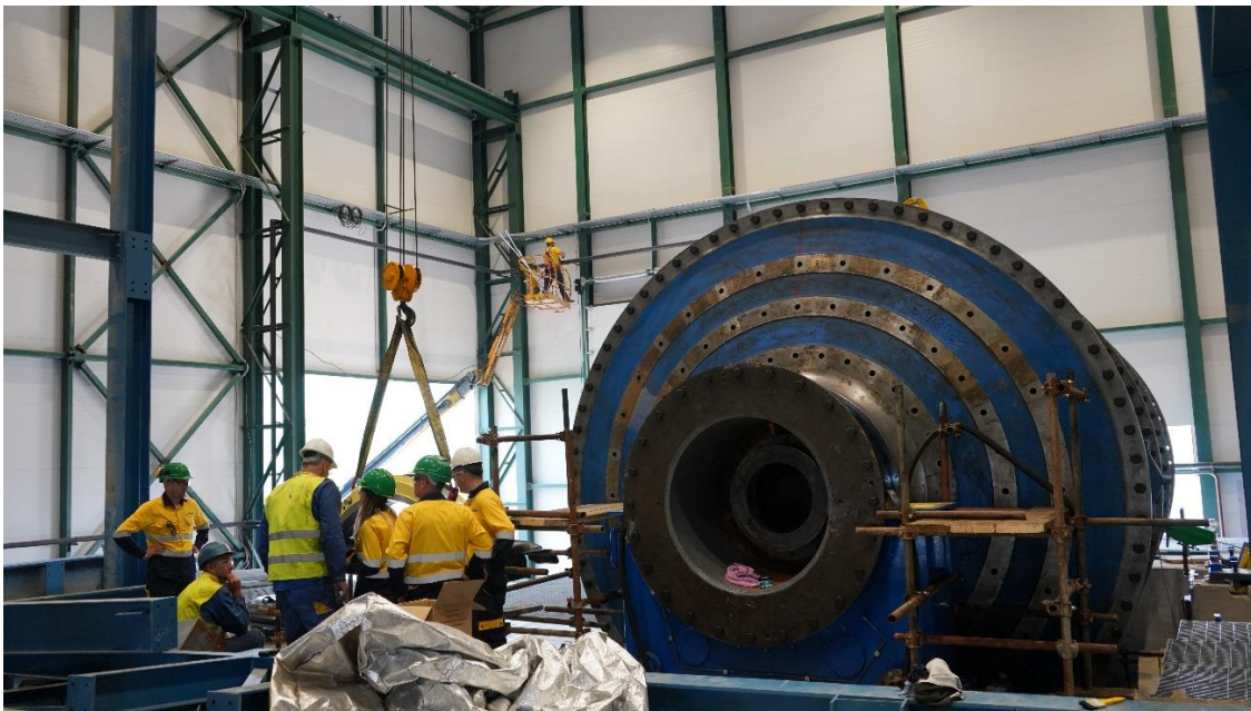
Figure 7: Ball mill, grinding building, July 2023
