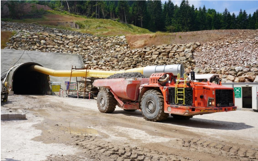
Figure 3: Lower Decline Portal
