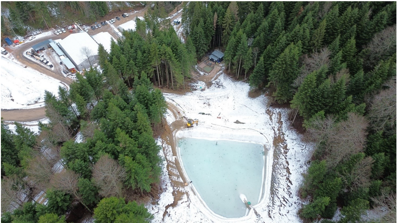
Figure 7: Water Treatment Plant, December 2023
