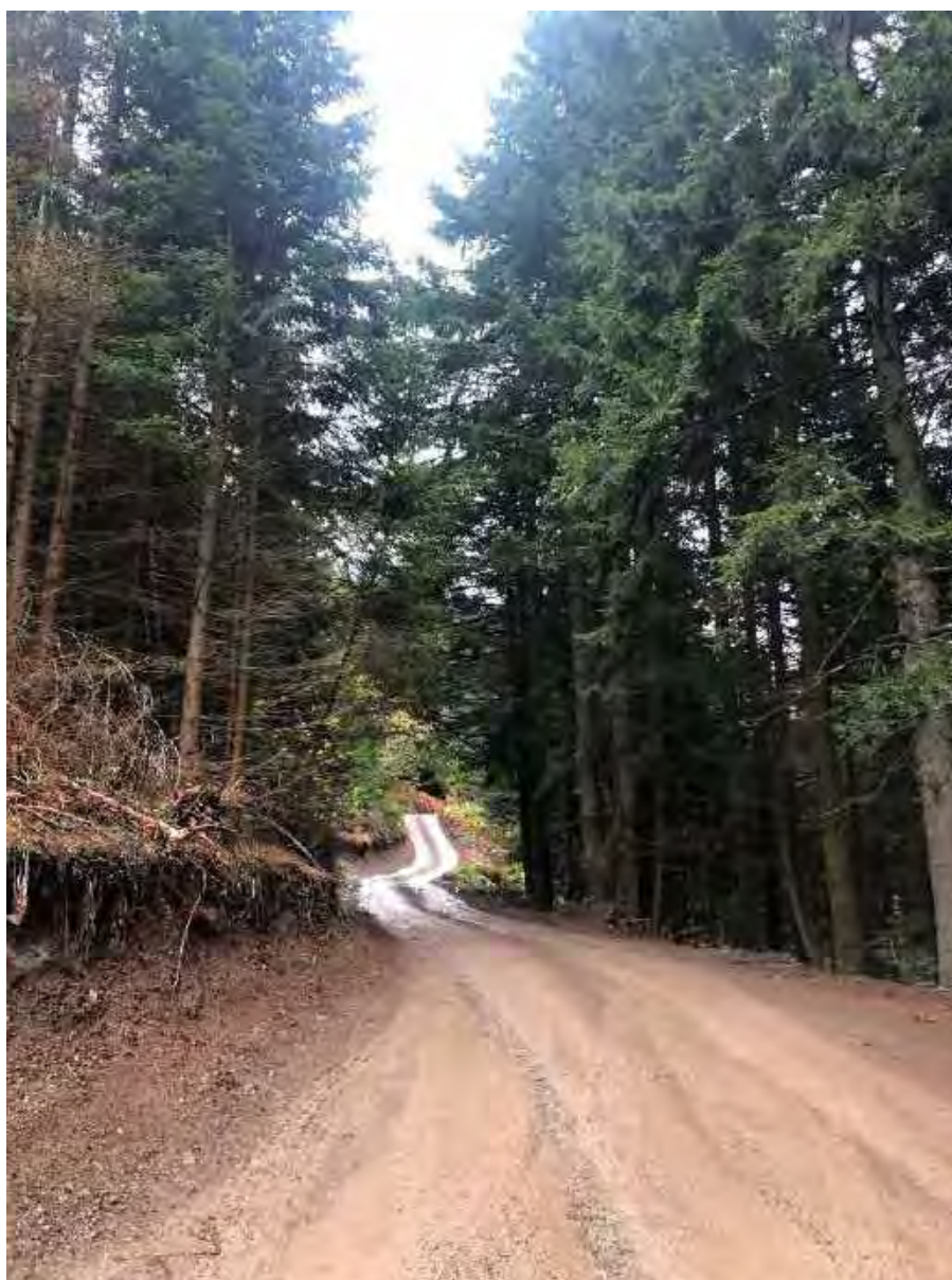
Photo 4.15.4: Typical Unsealed Forest Track
