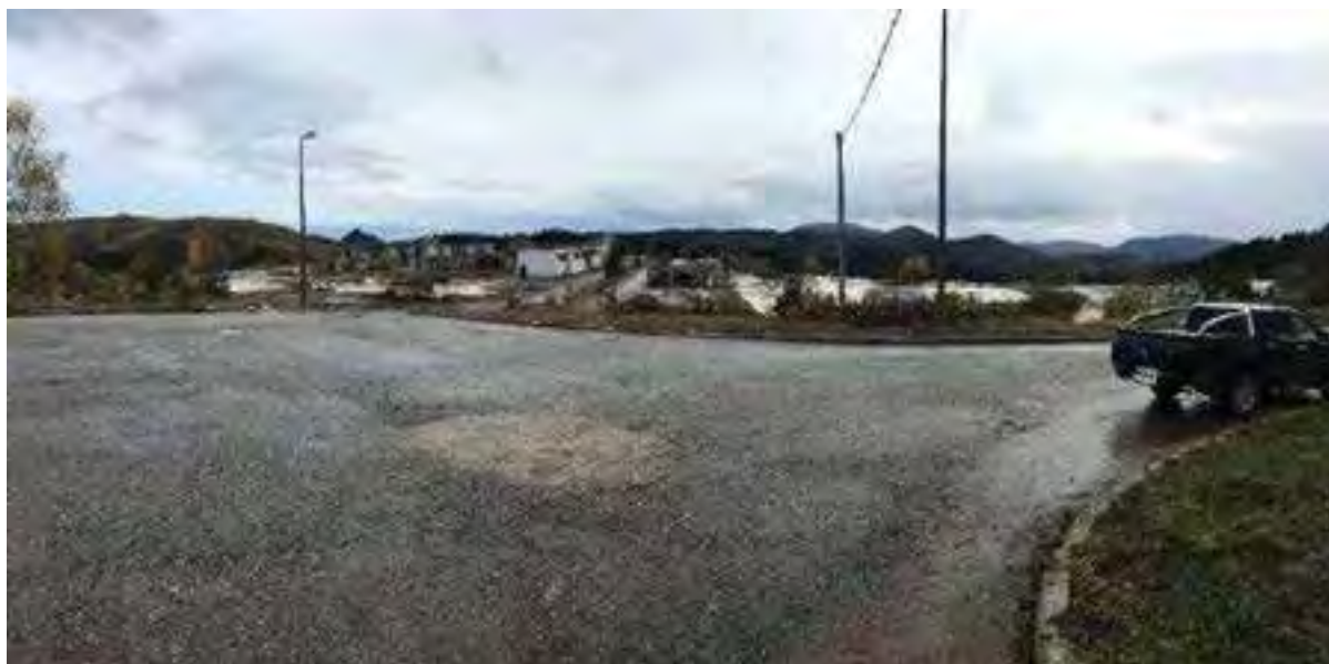
Photo 4.15.6: Remains of the former Vares Processing Plant (Pre-demolition)
