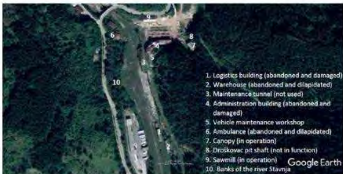
Figure 4.5.7: Surveyed Buildings at Droškovac Transfer Station, Vareš.
