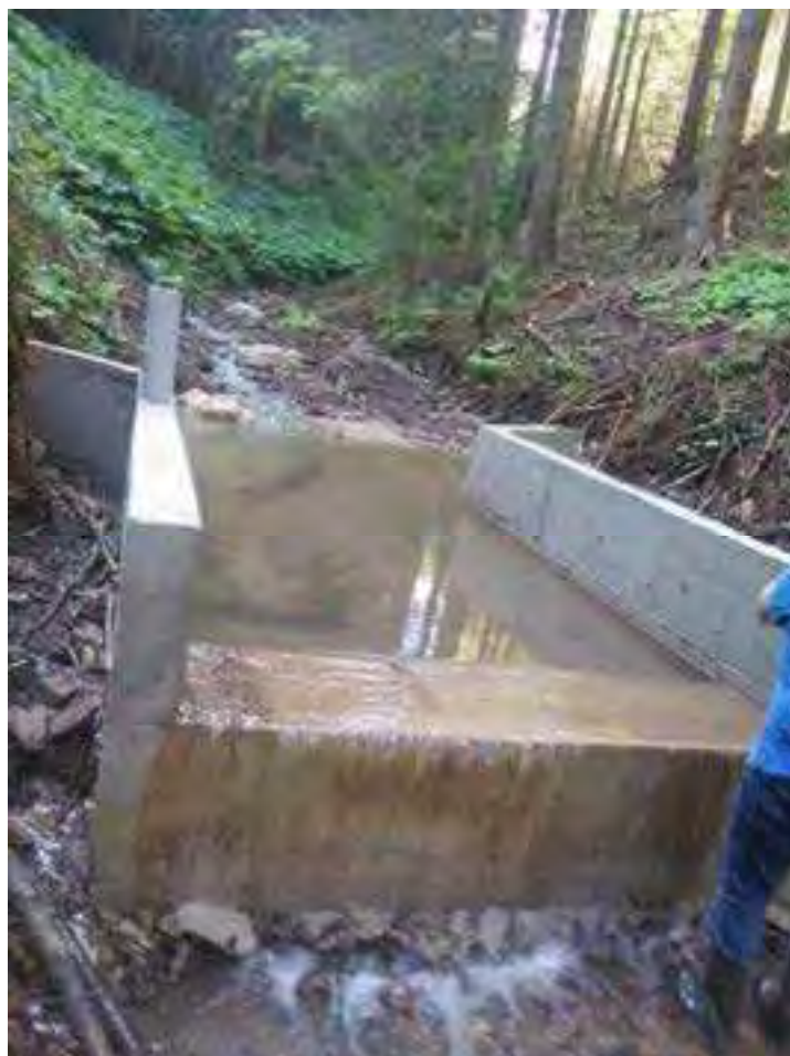
Photograph 4.9.2: Weir Installed Along Vruci Potak at PP-V.
