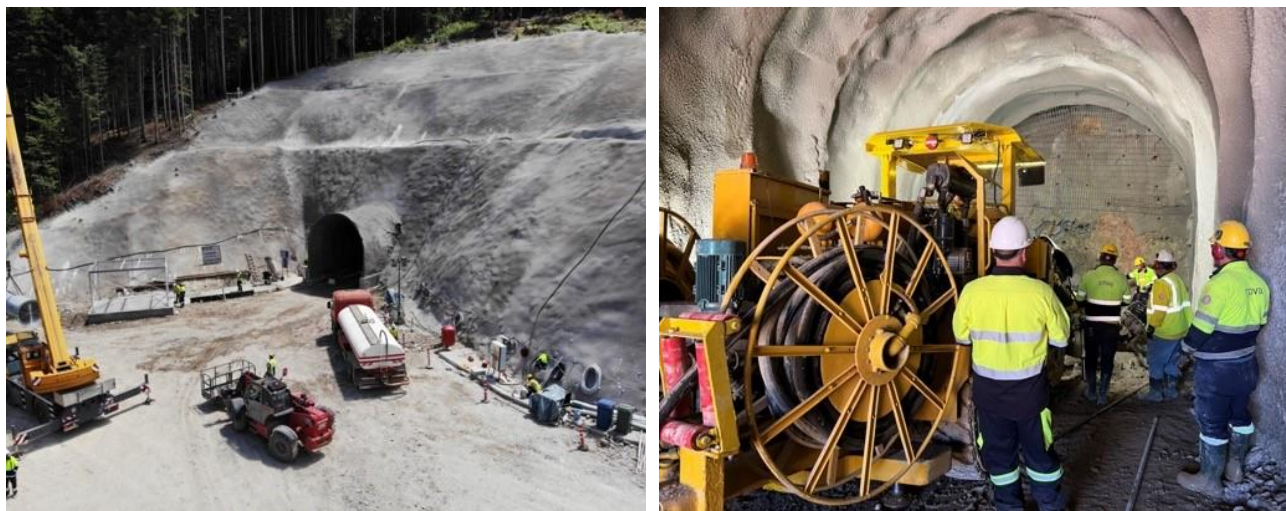
Figure 3: Lower Decline Portal and Underground Development (July 2022)
